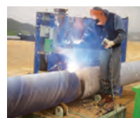
4. Steel Pipe + PHC Connection
