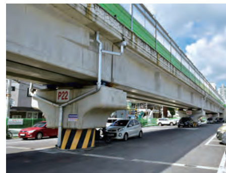
Kyengchun line, Mangu line, Jungwha elevated bridge L=21+2@30=81m, H=2.2m, B=6m
