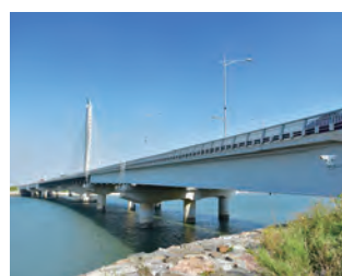
Incheon New Port, connecting bridge (2011) L=2@55+2@55=220m
